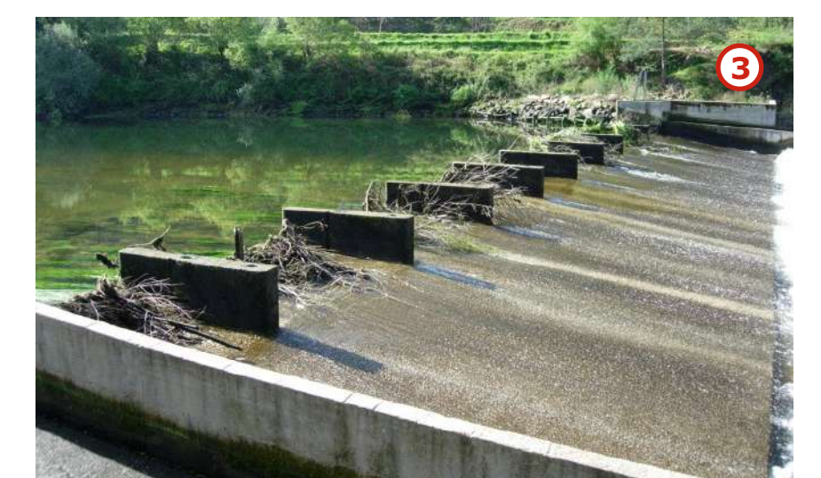
Designation: Louredo Weir Associated Uses: Leisure and recreational activities Adopted Solution: Natural fish pass
