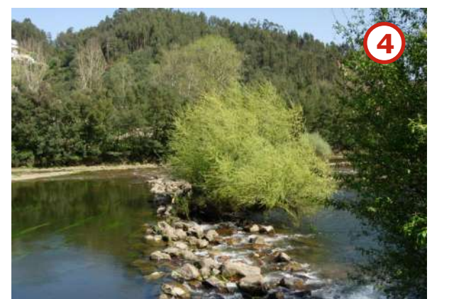
Designation: Ronqueira Weir Associated Uses: Old water abstraction for human consumption Adopted Solution: Removal
