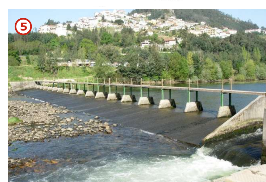
Designation: Reconquinho Weir Associated Uses: Leisure and recreational activities (bathing waters) Adopted Solution: Technical fish pass
