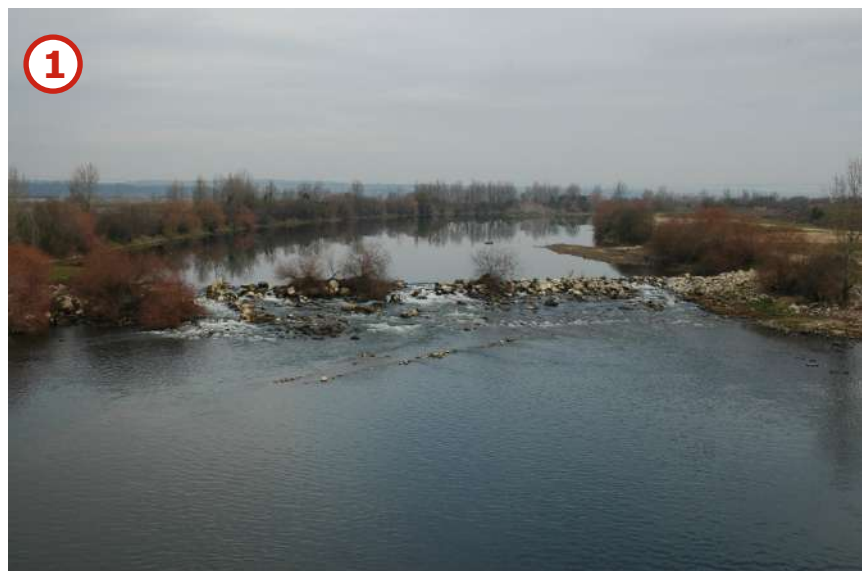
Designation: Formoselha Weir Associated Uses: Water abstraction for irrigation and industry, leisure and recreational activities Adopted Solution: Natural fish pass
