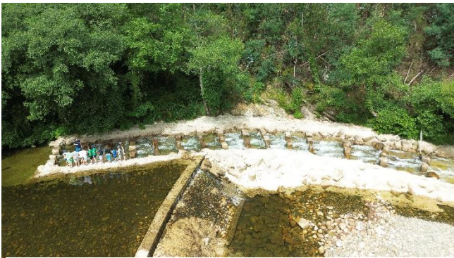
Naturalized fish passage (ramp), aerial view, Águeda river | © Esmeralda Pereira - University of Évora/MARE, 2024
